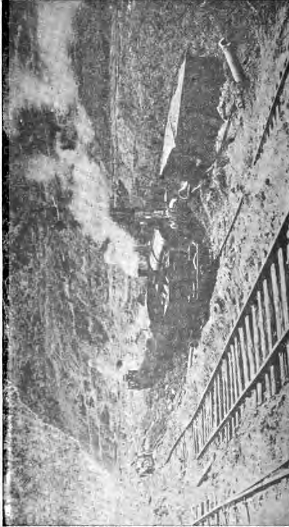
Steam Shovel loading a train of cars in Colobra Cut, Panama Panama-American & P. O. R. Mass. Agency & Advertising Bureau of New York
